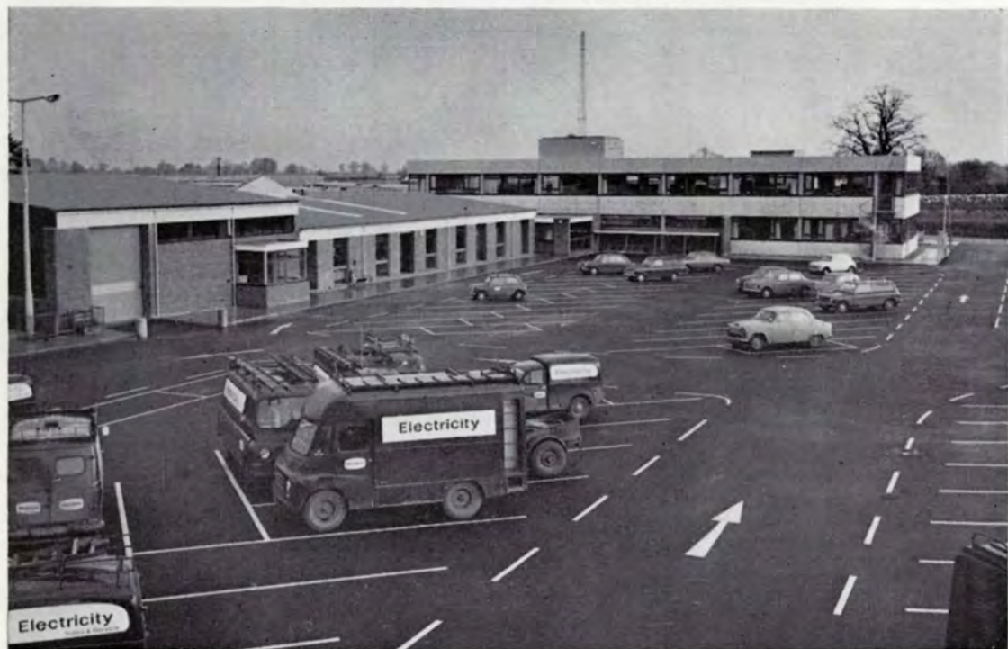
At the rear of the new office block, showing the stores and workshops and ample parking space for vehicles.
